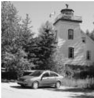
Janet Head Lighthouse showing overgrowth.
